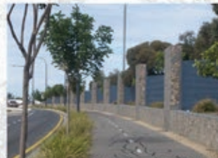
Infrastructure: Hallett Cove Noise Walls
